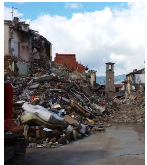
The main road through Amatrice in Italy in early October 2016, after the magnitude 6.1 earthquake in late August 2016.
